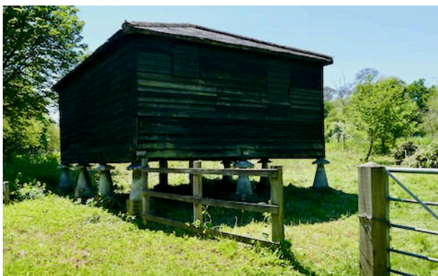
Clearance around the old Granary
